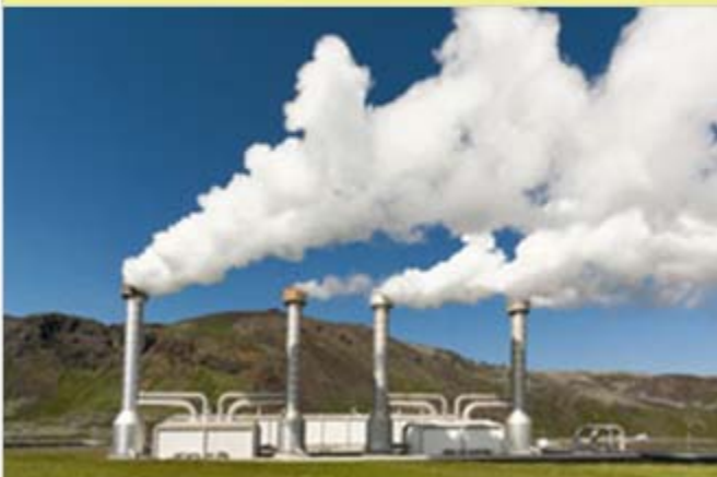
A Geothermic Power Station
